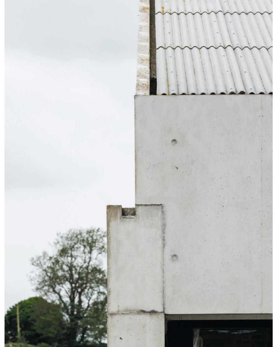
The corrugated fibre cement sheets are framed by the wall slabs of the gable and the eaves, giving them aesthetic support. The corrugated sheets of fibre cement structure the gently pitched roof, they intentionally stand out only slightly from the rest of the building.
