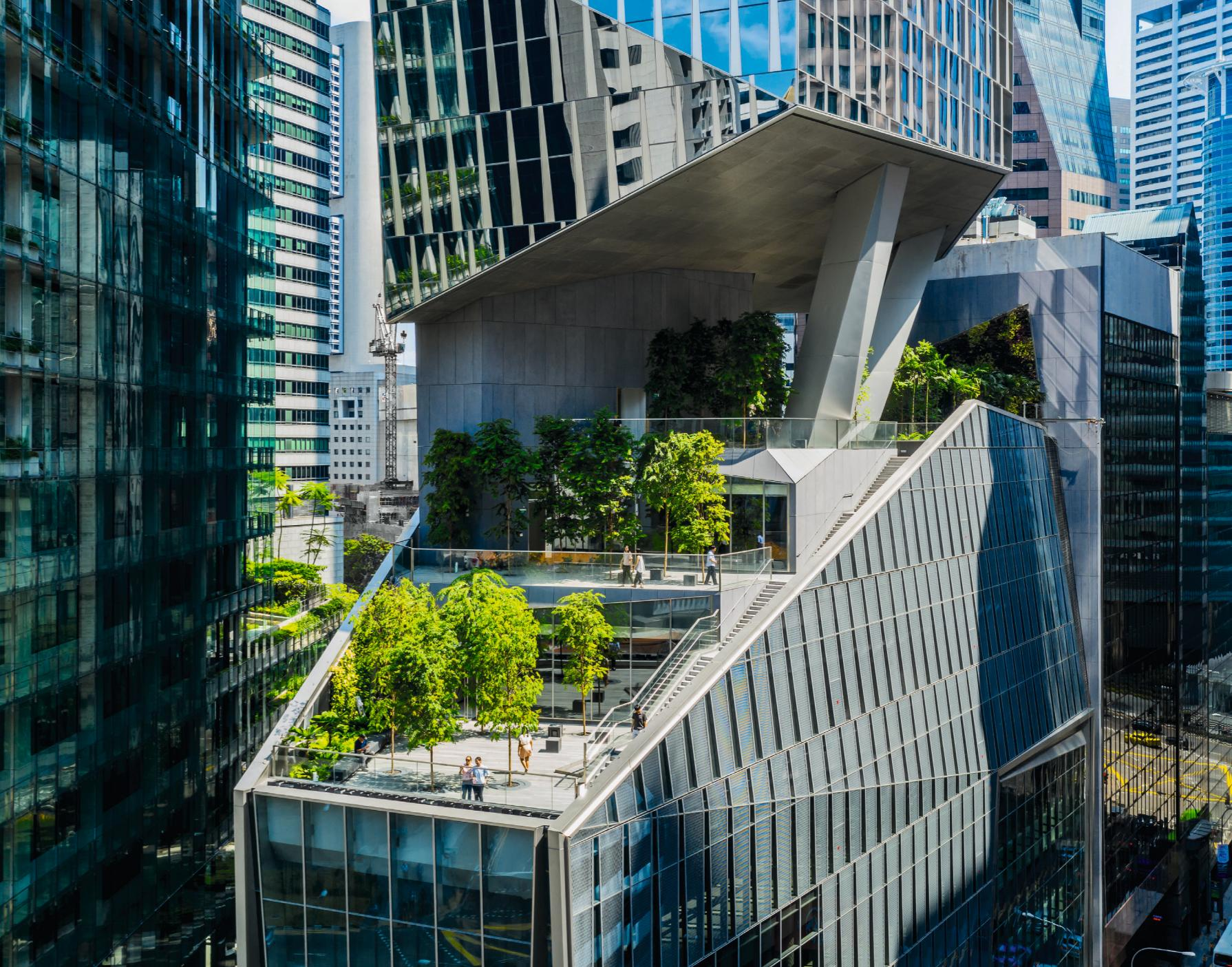
The tall office tower rests on three elements: two raking columns and the massive circulation core, which functions as the starting point for the angled, fibre-cement-clad soffit to the tower.
