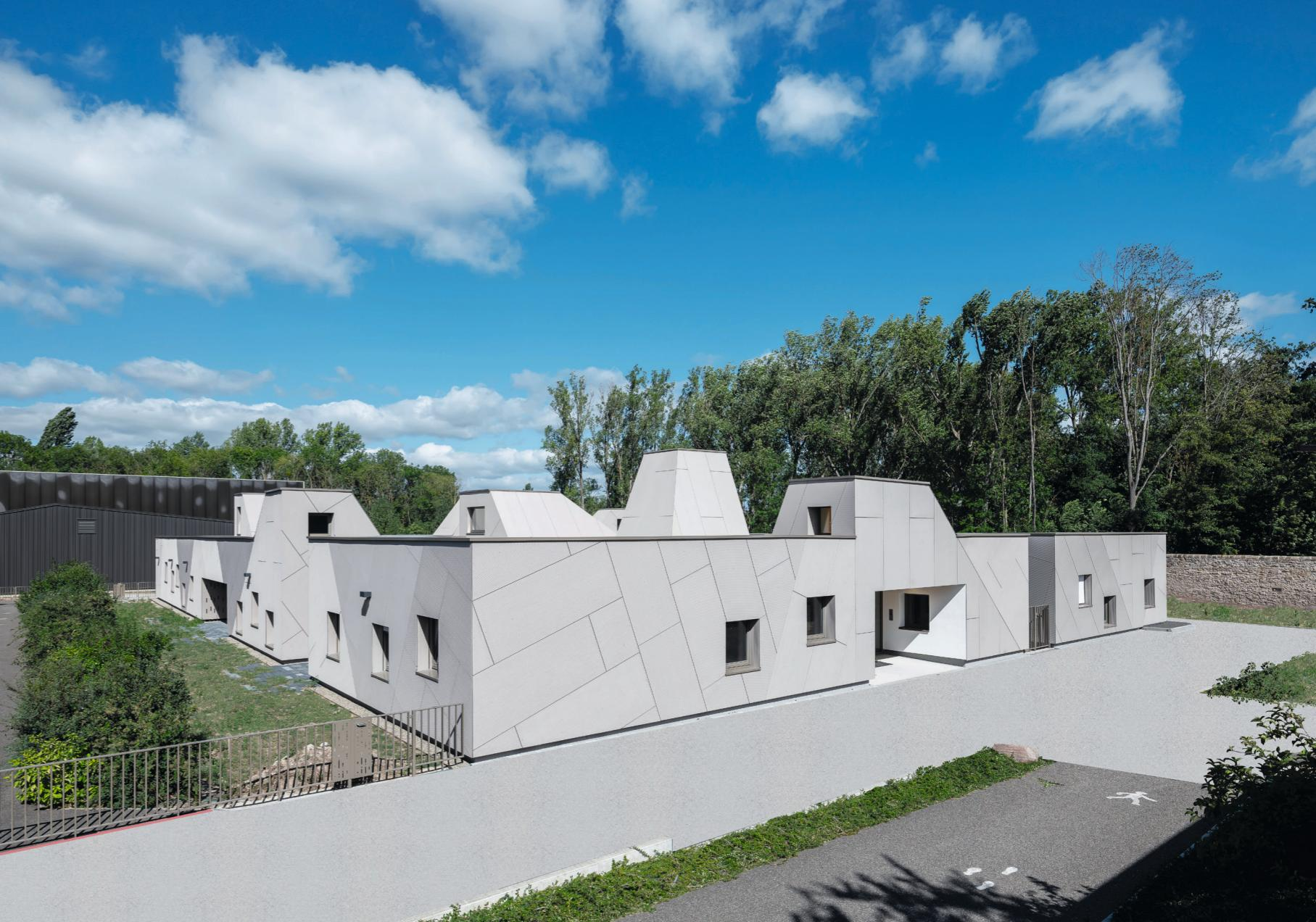
While the floor plan shows a clear structuring, in the section, elevations and in the perspective one recognises a game played with rooflights of different heights, which are accentuated by the way in which the scored fibre cement panels are mounted.
