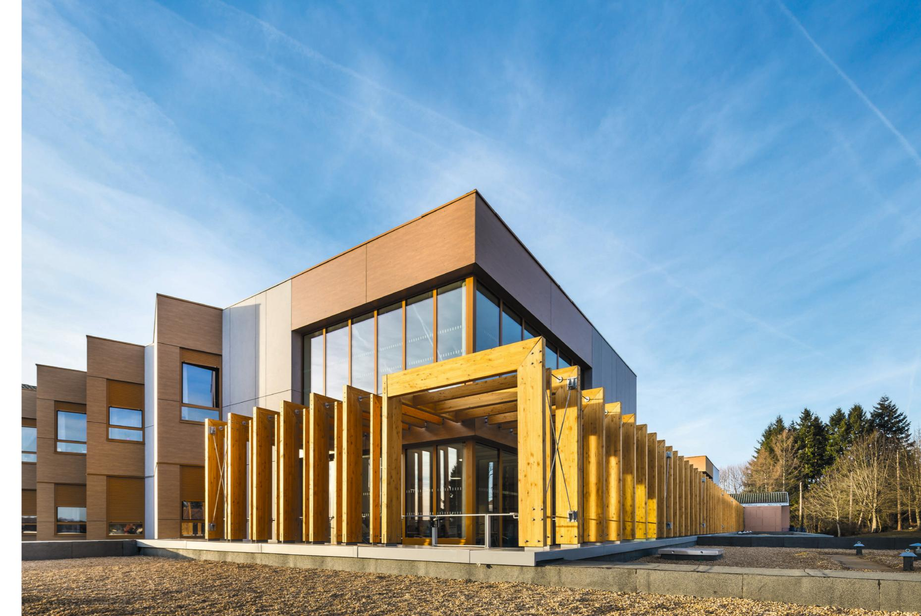
The middle courtyard is both the main entrance and new centre of the complex. It is the principal circulation space and its character is shaped by elements that are swivelled out of the facade, whose long sides are clad with fibre cement panels.
