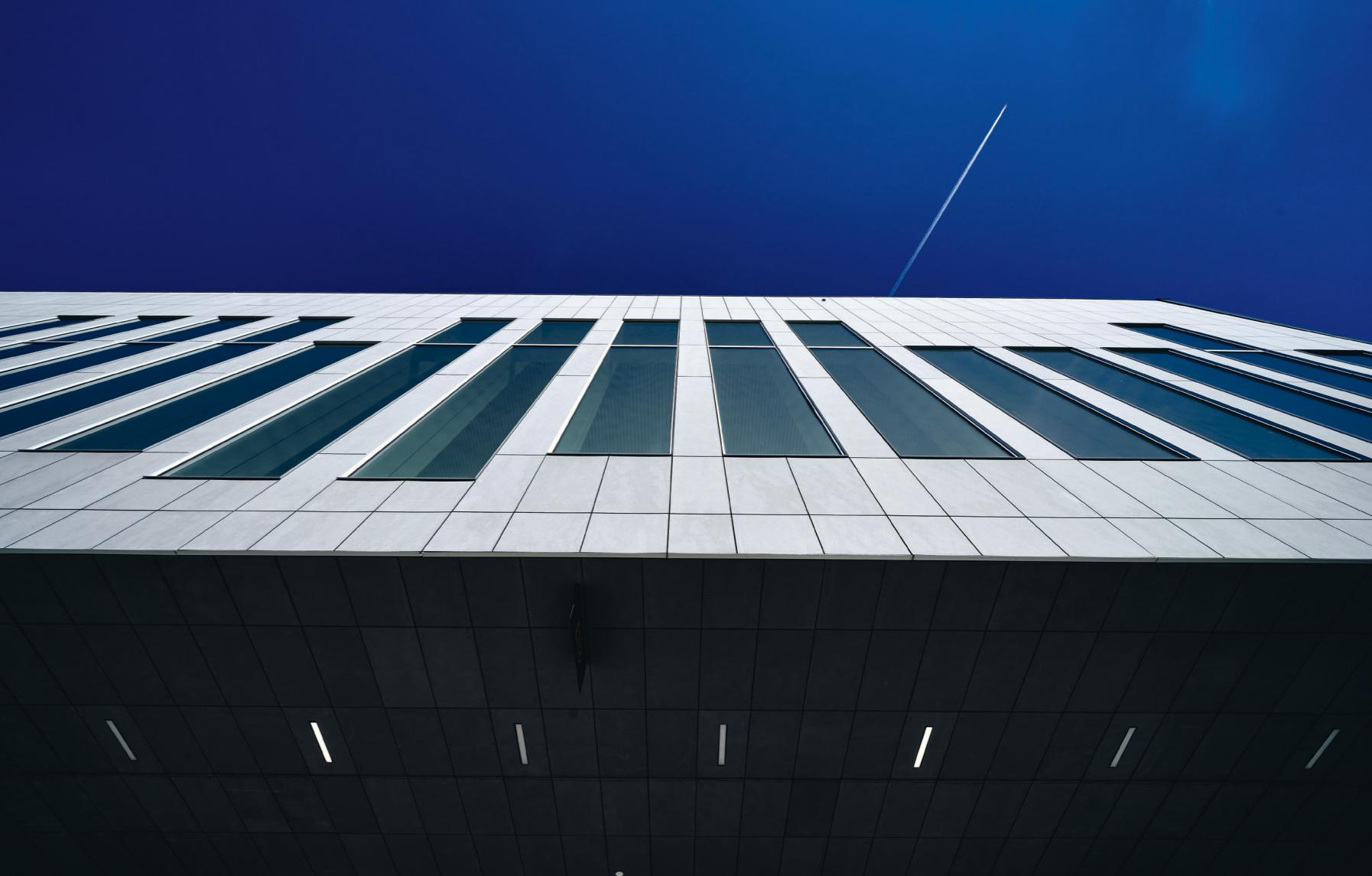
The straightforward quality of the interior is continued outside with an impressive precision. The soffits of the cantilevers are clad with the same kind of fibre cement panels, continuing the pattern of joints up to the glazed front to the ground floor.
