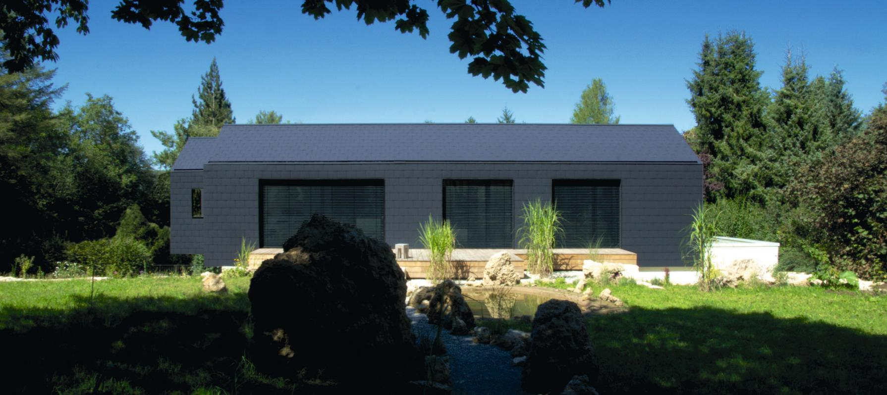
The sizes of the windows were adapted to suit the dimensions of the fibre cement slates, in this way minimising waste. In addition, the windows have a slightly projecting metal reveal that provides a simple form of sun protection.
