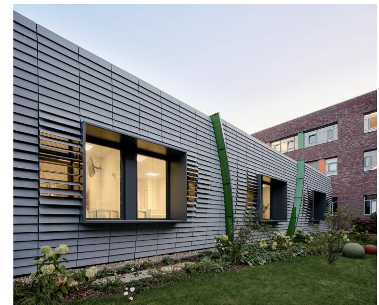
In terms of colour the green-painted glass fins refer to the neighbouring buildings and intentionally interrupt the façade. The generously sized windows to the single rooms are partly covered by the facade. Where the angle at which the light grey fibre cement louvers are mounted changes incrementally, row by row, to an almost horizontal position, an effective visual screen is created, while still allowing daylight to enter.
