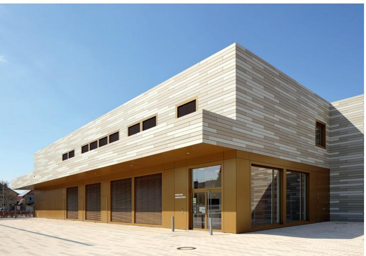
The building's elongated form played a decisive role in the design of the facade. Using long, narrow fibre cement panels three metres long by 18.5 cm wide, in three different shades of beige, a sample mounting plan was made so that, from the start, the pattern of the joints could be carefully controlled. The result is an extremely precise facade, worked out in detail down to the smallest corner.
