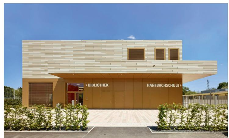
On the entrance side of the building there is a generous canopy roof and the facade is divided into two parts: while the ground floor has bronze-coloured metal elements, on the upper floor the fibre cement panels begin, which are in different shades of the same colour and were mounted with the vertical joints staggered in each "course", which emphasises the horizontality of the building.
