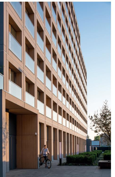
The panels of fibre cement were cut precisely to the width of the box-like windows; at the top there is a narrow parapet flashing that allows rainwater to run off optimally.
