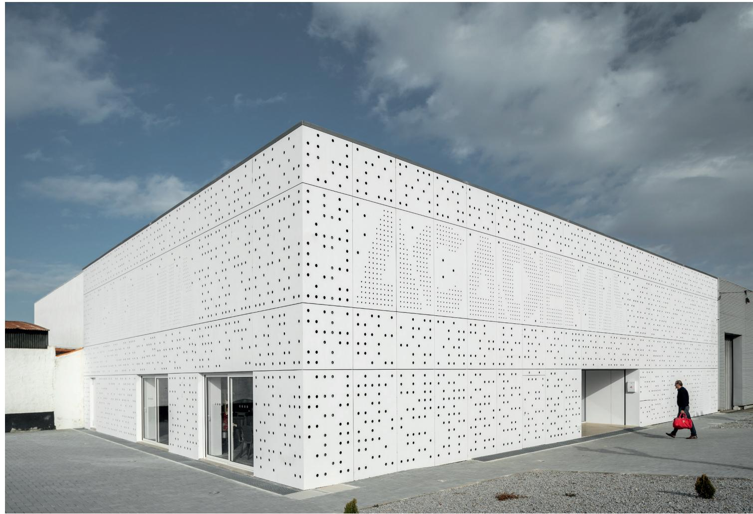
Like in the interior, the panels of fibre cement are pure white in colour. For the perforations and the pattern of the joints, it was very important that the fibre cement panels be through-coloured to avoid creating conspicuous edges around the circular holes.
